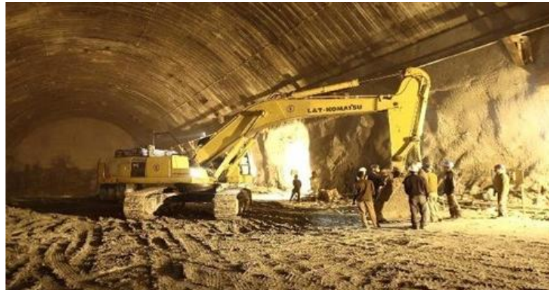
Srisailem HE Project - Andhra Pradesh (900 MW) Largest Underground Cavern in Asia 25.7m (W) x 53m (H) x 236m (L)
