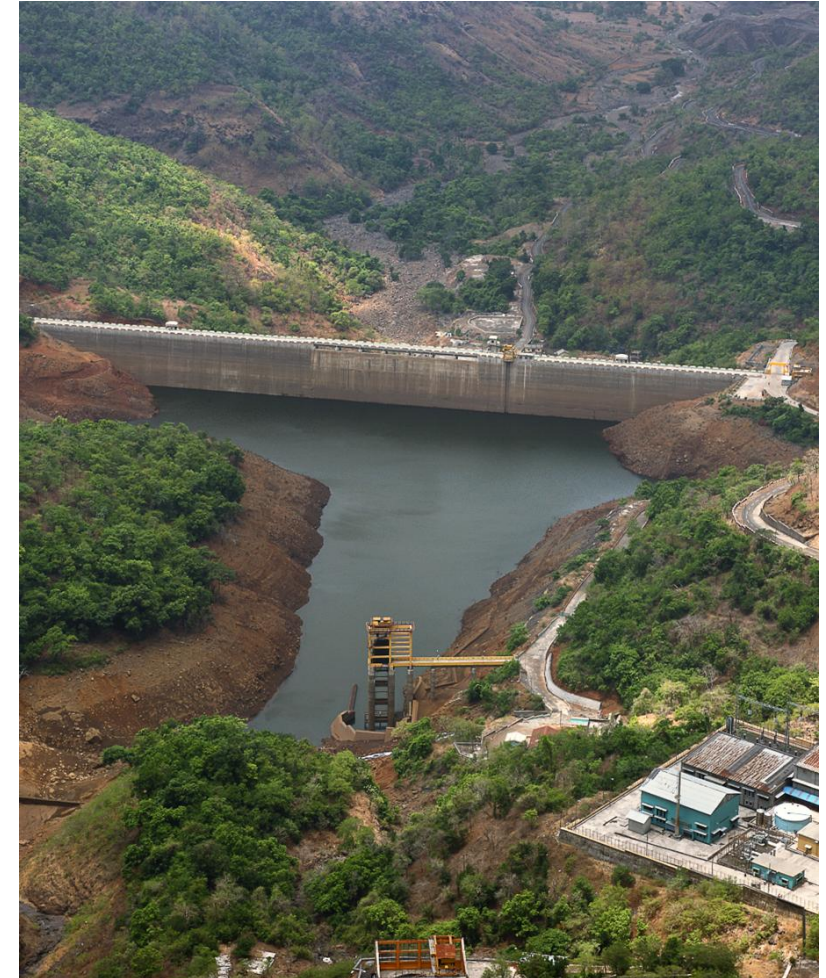
Ghatghar Dam - Maharashtra 84m high 10th fastest completed dam in the world & India's first RCC Dam
